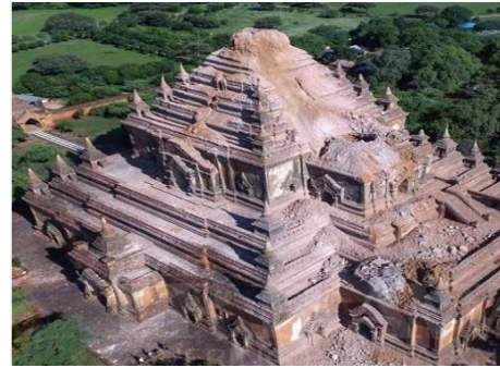
Figure 5. One of the Damaged Pagodas, Bagan, Myanmar
